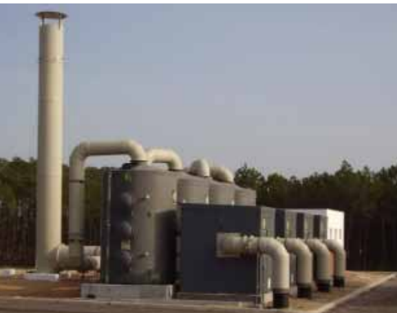
Deodourisation at urban WWTP with a double carbon bed tower for 40.000 \text{ m}^3/\text{h}
