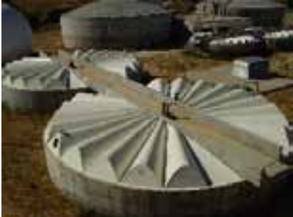
Circular cover for decanter with intermediate bridge
