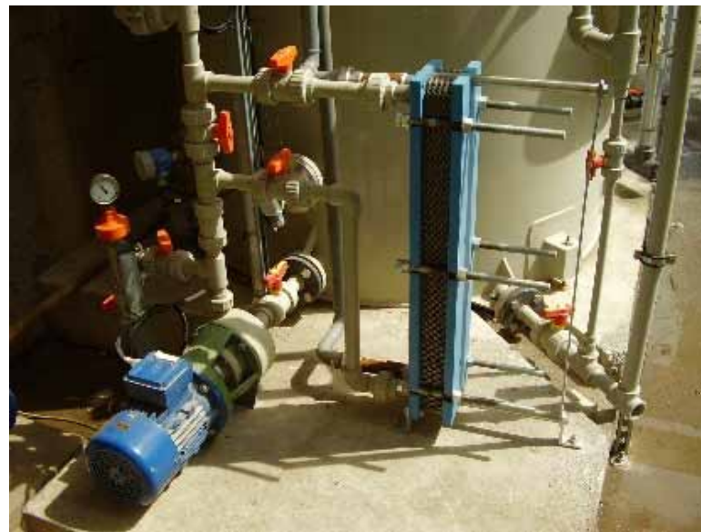
Transfer pumps to transfer to consumption points
