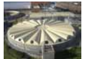
Decanter biofilter circular cover
